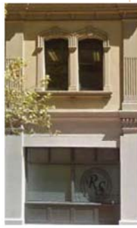
Brick Faced with Stucco historical facade only (Former 'Hawken & Vance Produce Exchange') 1883
