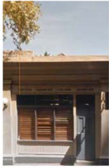
Face Brick + Render with tuscan pilasters (Former 'Royal George Hotel' / 'Cuthbert's Patent Slip') 1903
