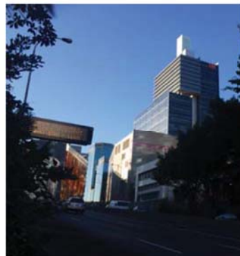
WESTERN DISTRIBUTOR VIEW NORTH
